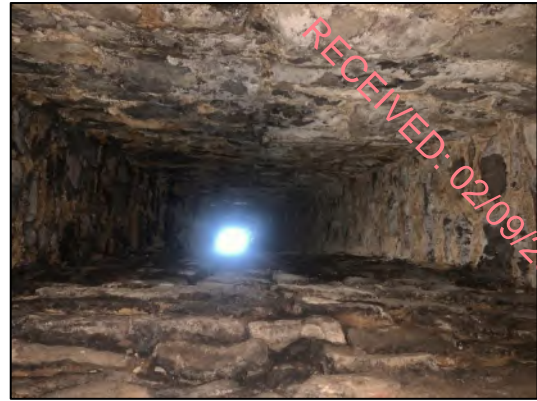
Plate 4-12 Chimney stack – Possibly hiding cracks or crevices
